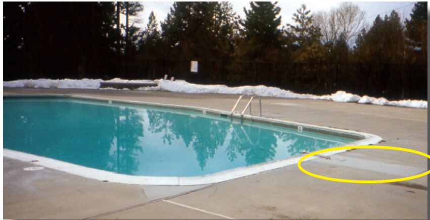
Pad where diving board used to be located. Air gap has been eliminated
