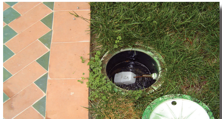
Swimming Pool: View of automatic float control valve
